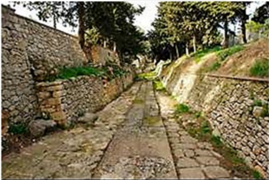
Streets with paved roads including rainwater drains
