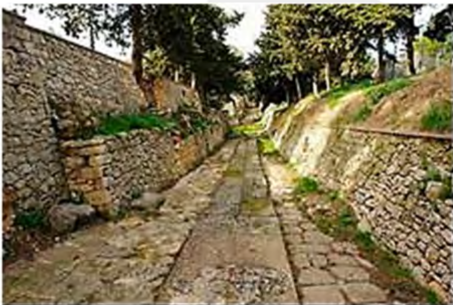
Streets with paved roads including rainwater drains
